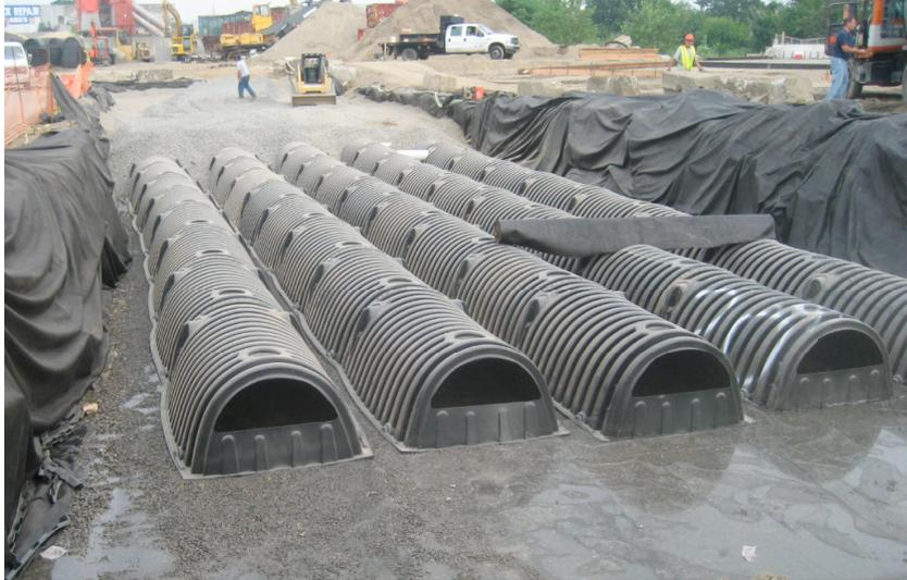
By enhancing tree pits with StormChambers, or similar structures, every 25-foot length of adjacent roadway would have a storage capacity of about 2,000 gallons of water. The Mayor's plan to plant a million trees, if coupled with below ground storage, as described here, would have a stormwater storage capacity of two billion gallons; roughly one-tenth of the annual total combined sewer overflow.
